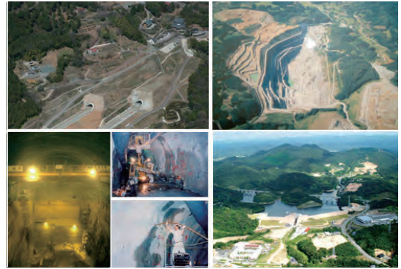
Tunnels, rock slope, underground powerhouse, and dam
