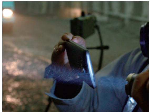
Dust monitoring using a mobile phone at a tunnel construction site
